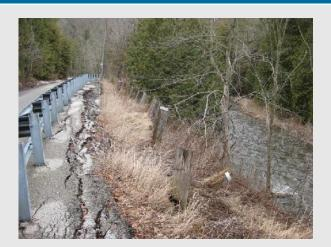
Evidence of toe erosion was observed at several locations where the road was close to the watercourse. The watercourse position appeared to be stable suggesting that the removal of fine bank material was replaced by the slumping banks which in turn resulted in the road slippage.
