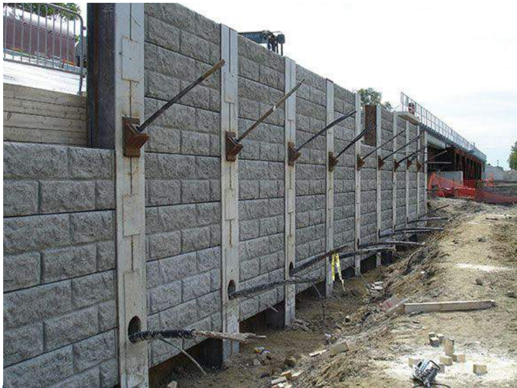
1 - Soldier Pile and Lagging System
