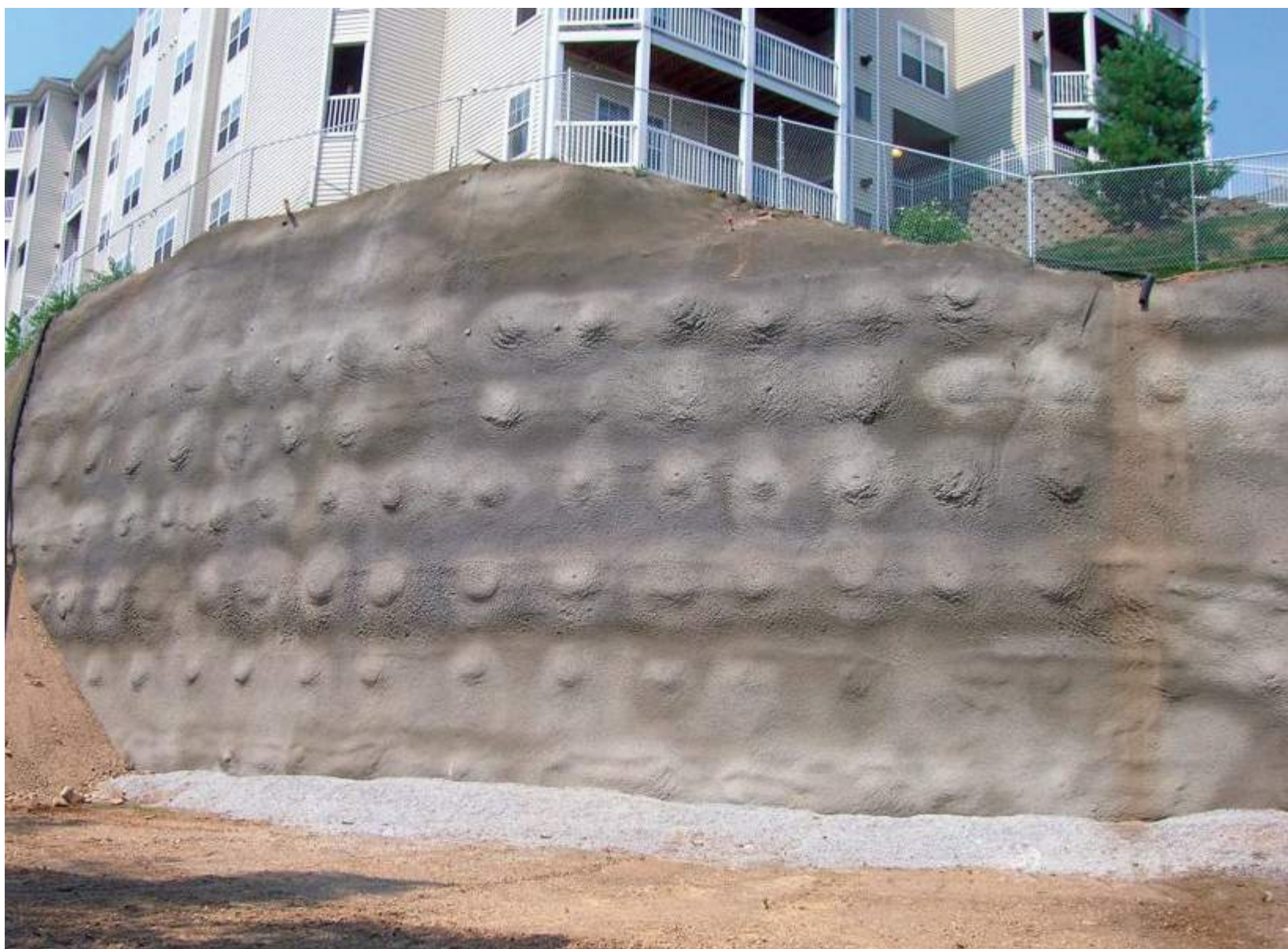
5 - Soil Nails/Micro-piles and Shotcrete Facing
