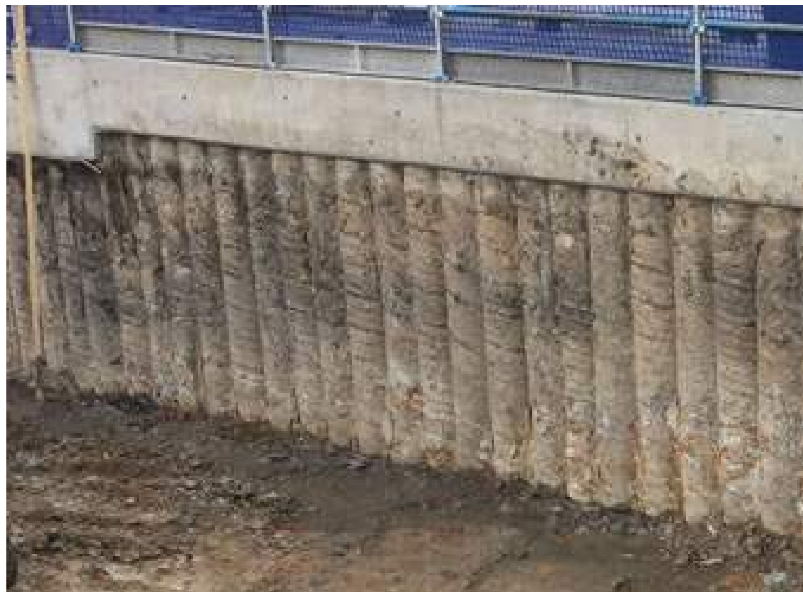
7 - Tangent/Secant Pile Walls
