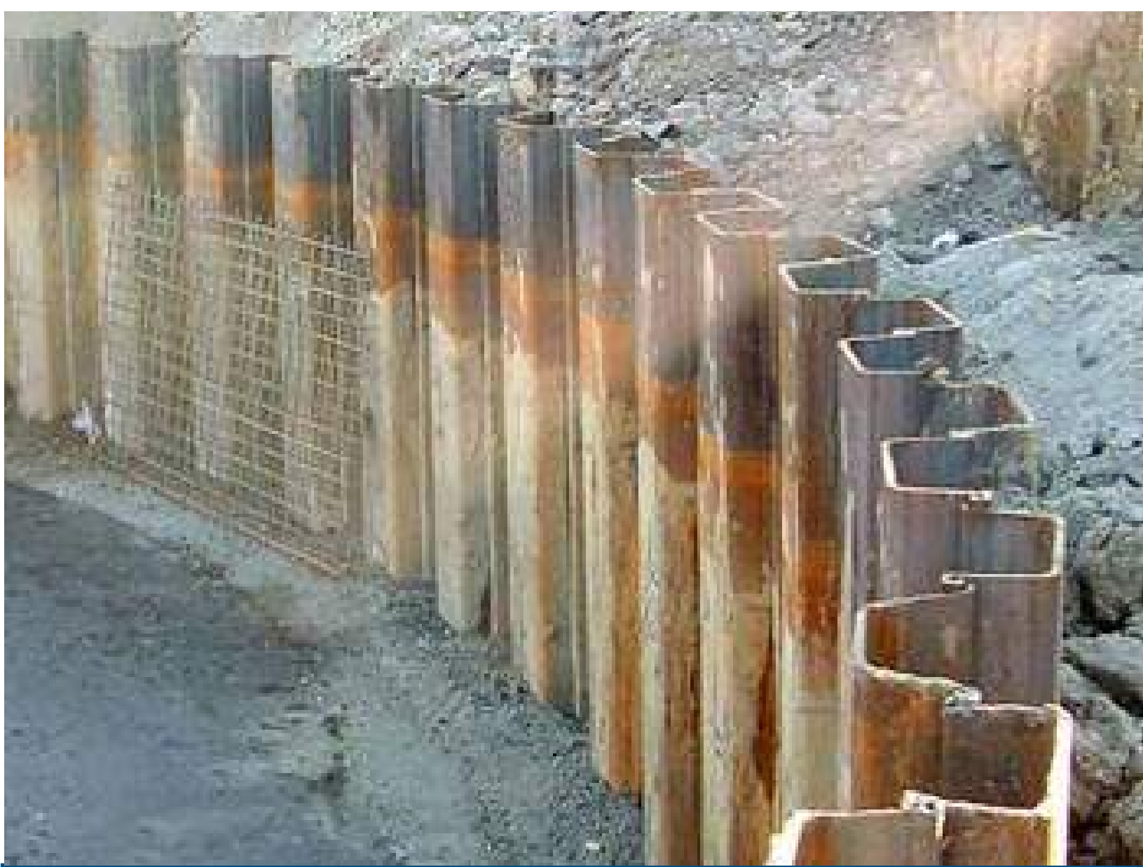
2 - Sheet Pile Wall
