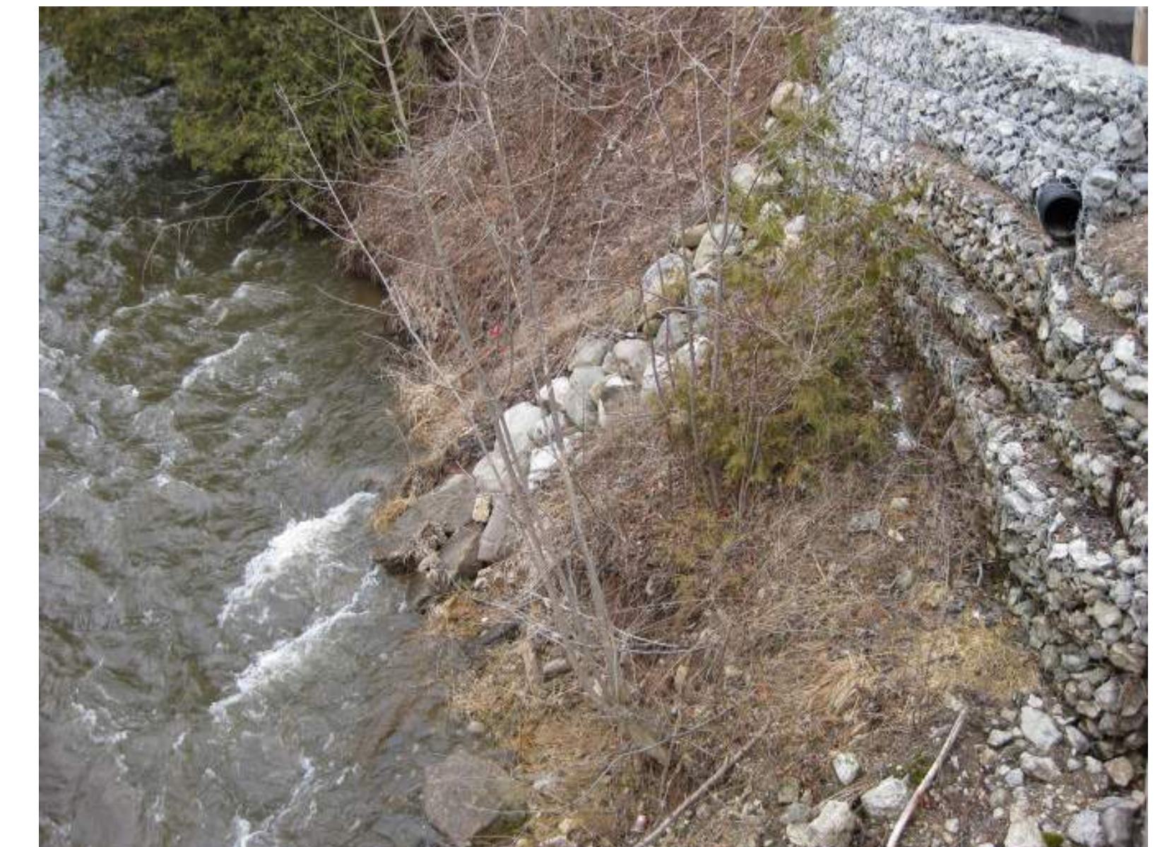
Gabion baskets, on bridge facing west
