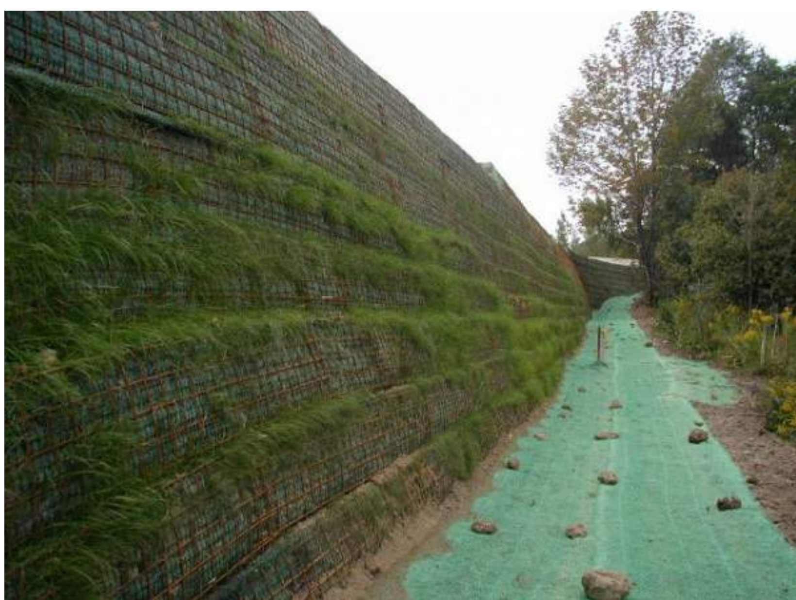
4 - MSE Retaining Wall
