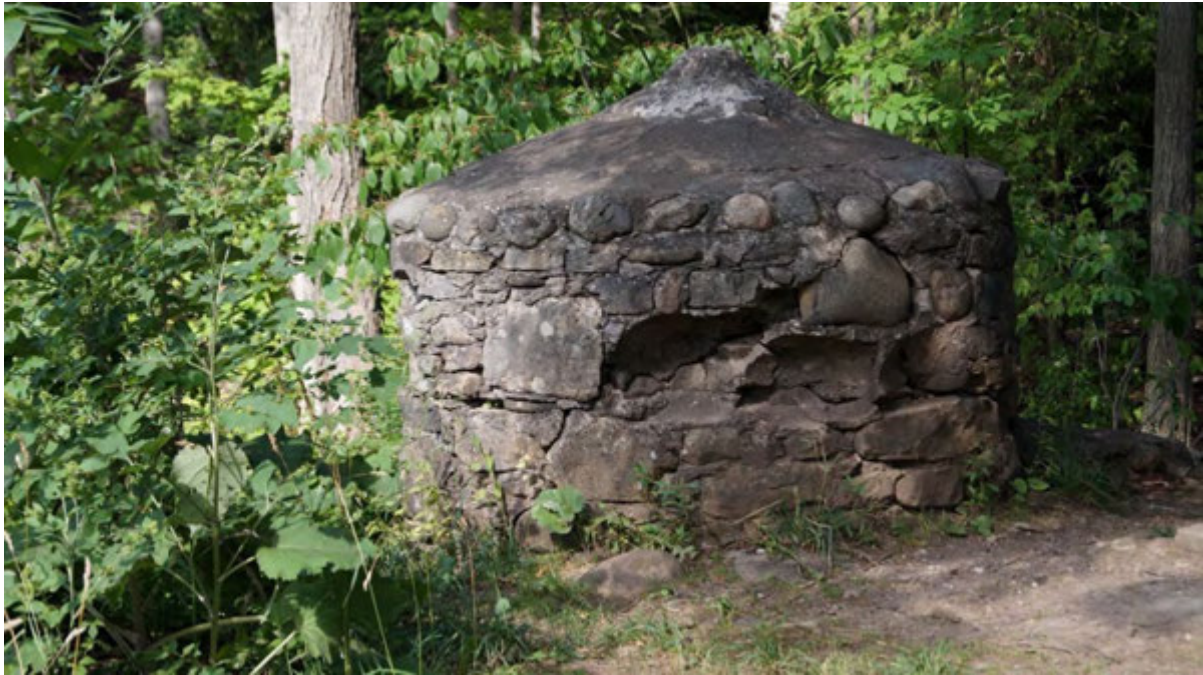
5. riverbank circular oven of stone blocks and cobblestones with an arch on one side and a concrete cap (arch opens to show a cavity inside)
