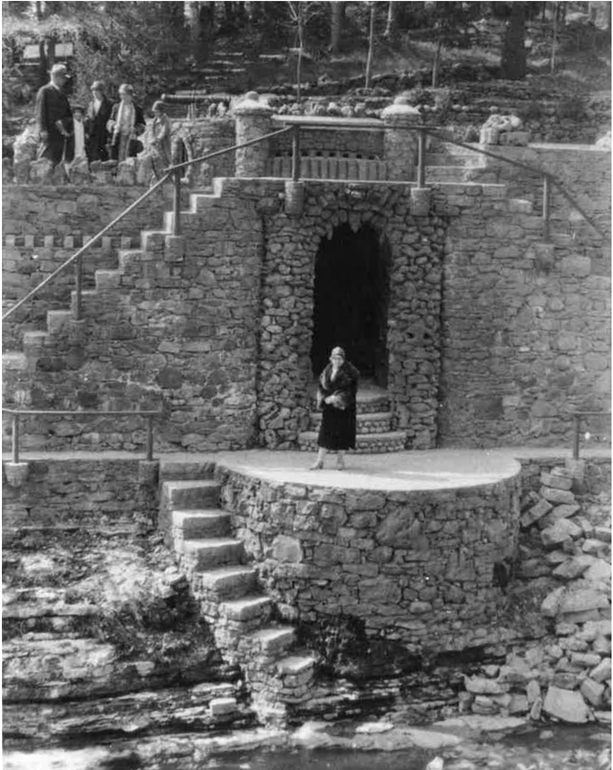
Yellowstone Cave, an elaborate grotto built into the high retaining wall beside the dam, was Mack's 1928 project. The photo reproduced by Credit Valley Conservation shows the grotto's three levels – a rounded bottom platform with stone steps down to the river's edge, a tall stone wall with a round-arched entrance into the grotto's interior, and a parapet roof on top of which a flower garden was planted.
