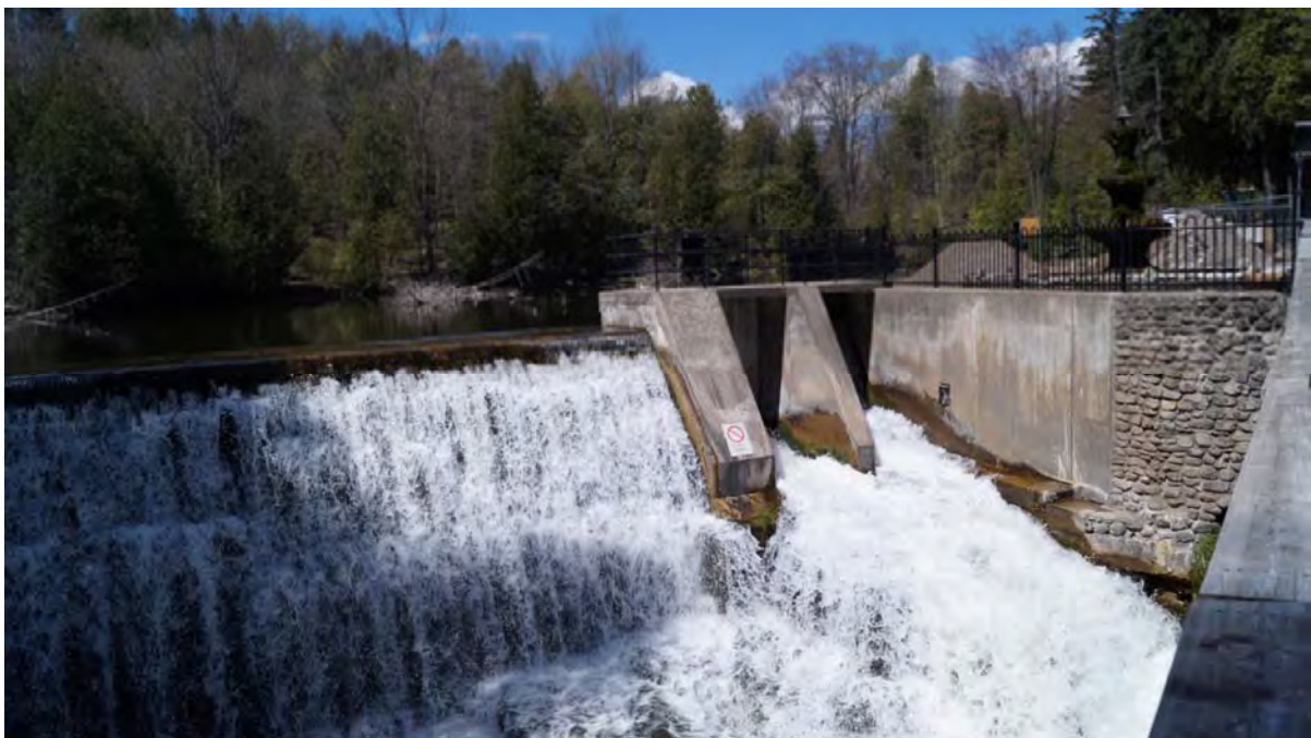
32. stone and concrete dam with stone cascades and concrete sluice way
