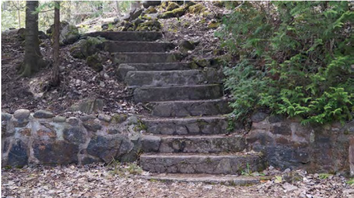
25. concrete-encased stone steps formerly leading to Bide-a-wee Cottage
