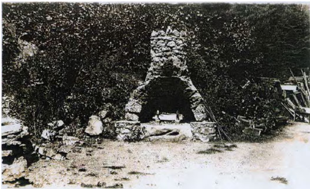
The photograph reproduced by Credit Valley Conservation shows another of the fanciful stone creations in Mack's Park. The fire pit employed the same rock-faced stone treatment used on other features. The pit's rounded platform and round arch were motifs seen elsewhere in the park. A massive chimney crowned the pit.
