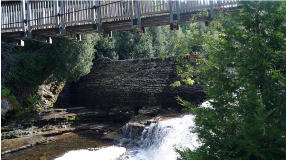
33. dam showing stone face at low river flow (note suspension bridge above)
