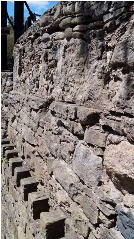
36. detail of stone dentils in the grotto's face
